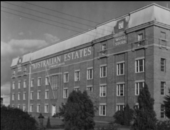
Australian Estates Woolstore Sunshine Road West Footscray. 1950
