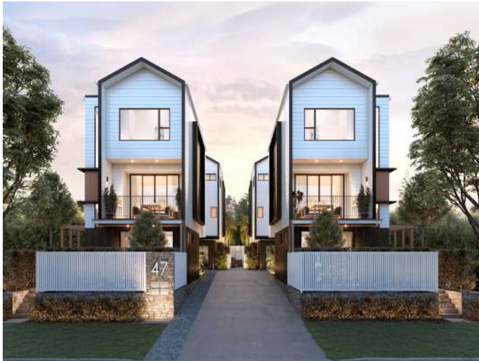
ST BARTS AT KINGSCLIFF
