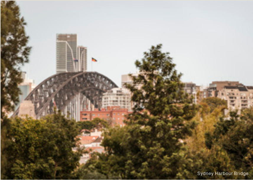
Sydney Harbour Bridge
