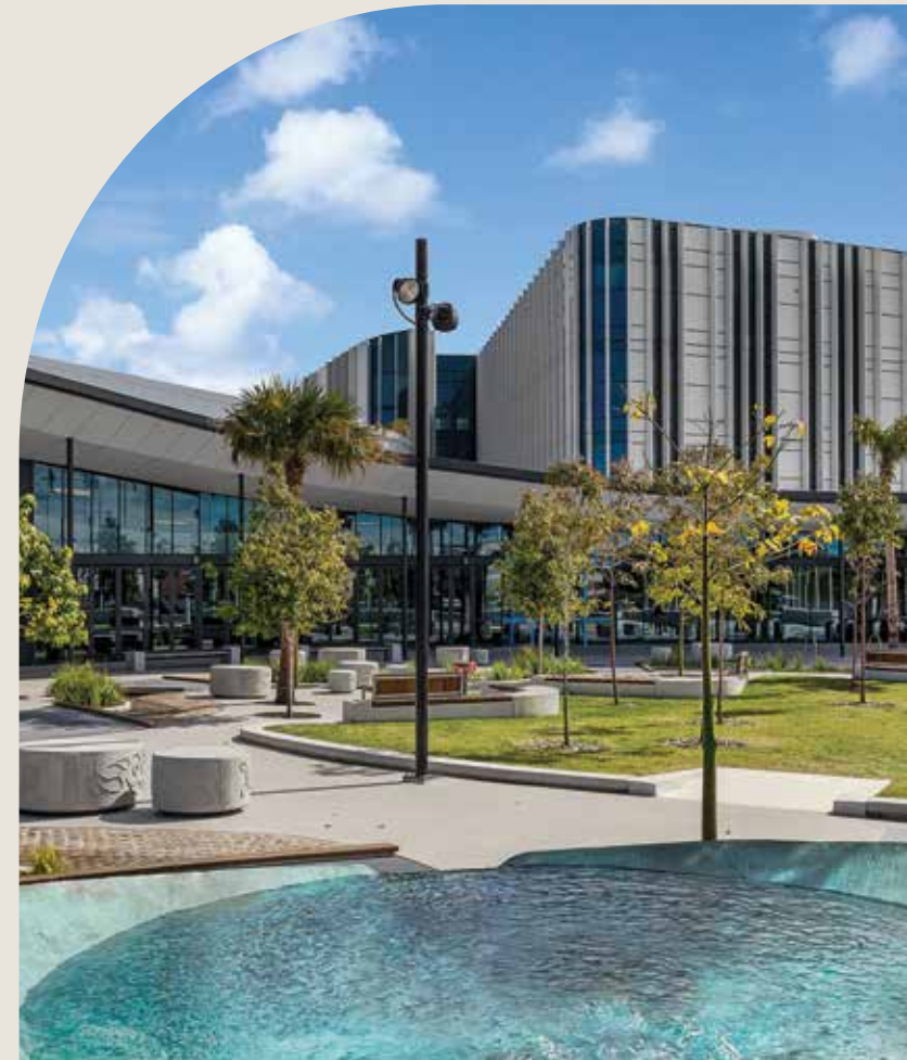
Shellharbour Civic Centre, NSW
